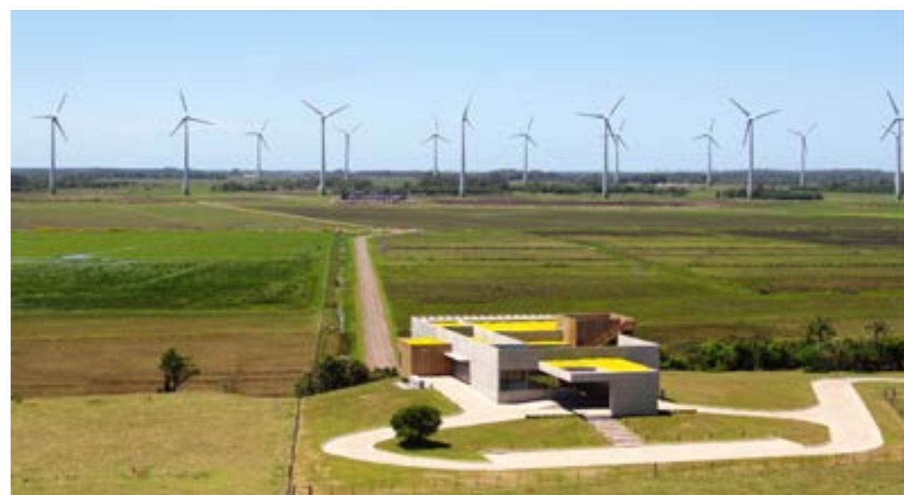
Wind complex at Osório, Brazil
