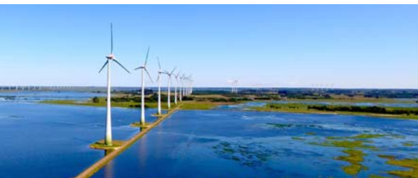
Wind complex at Osório, Brazil
