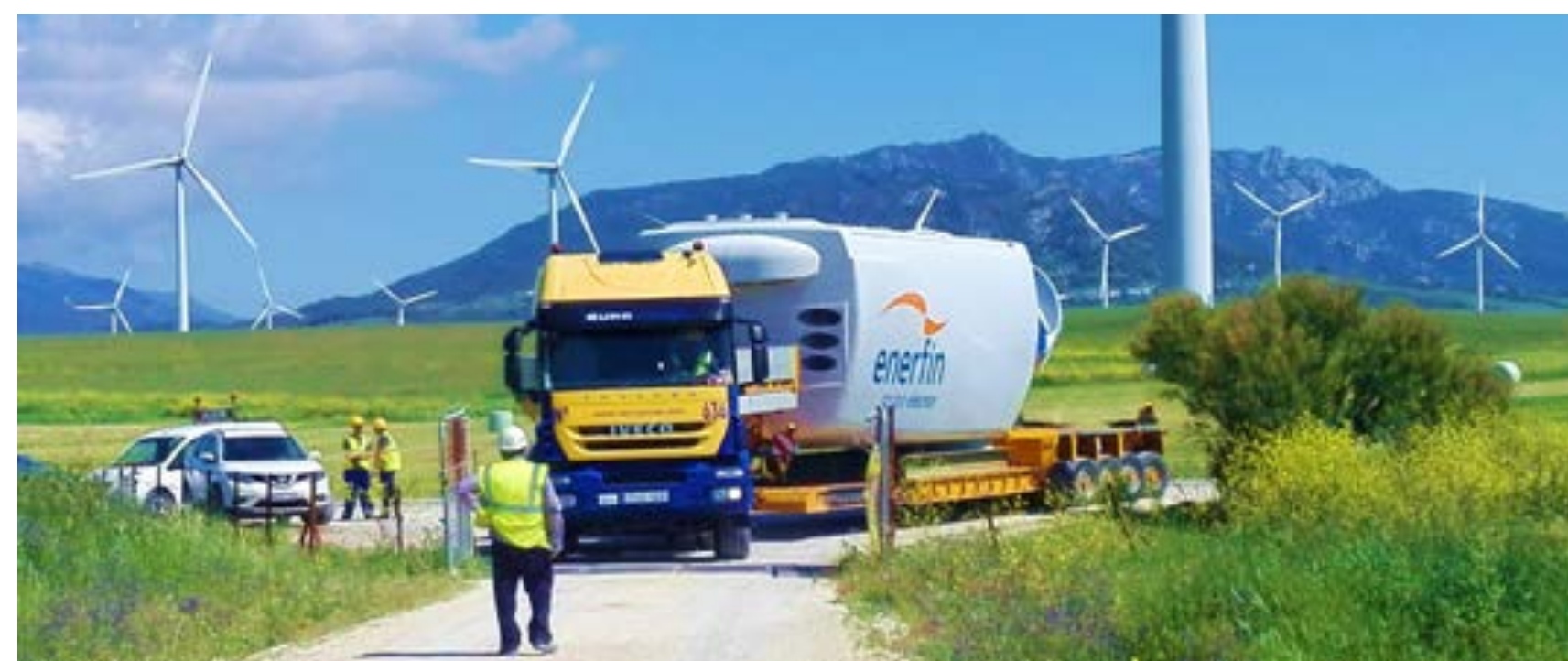
Wind farm construction. Cofrentes, Valencia
