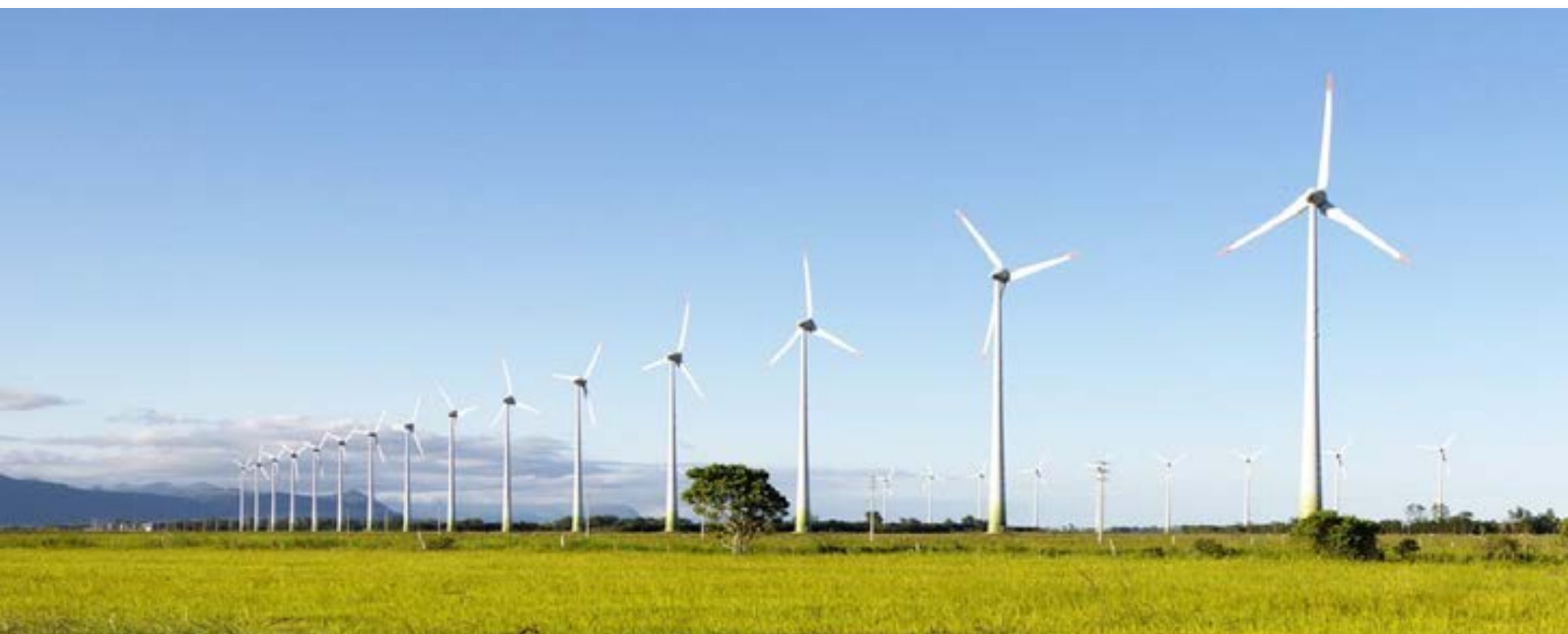
Wind complex at Osório, Brazil
