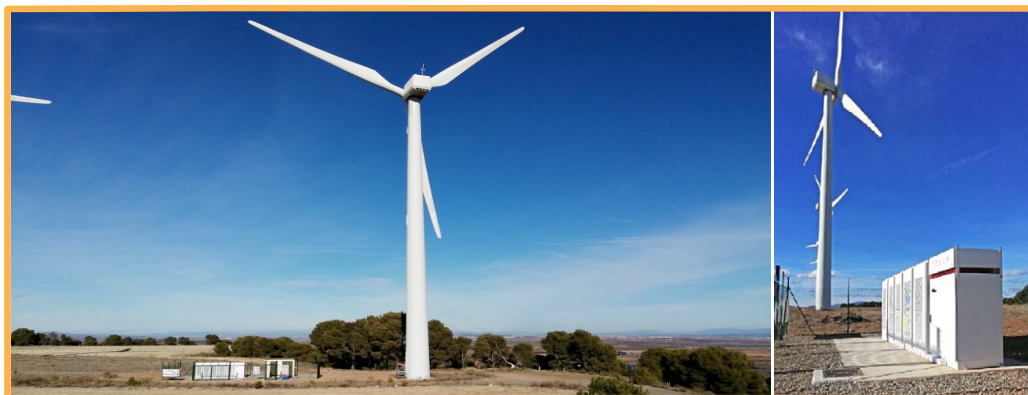
Storage system using Ion Lithium battery at P.E. Montes de Cierzo (Navarra, Spain)
