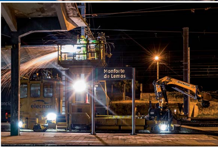
Refurbishment of overhead power line between La Rua Petín and Monforte de Lemos (Orense-Lugo)
