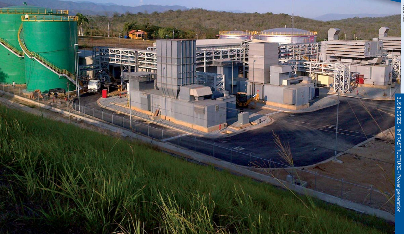
EDC-Sur thermoelectric plant (Venezuela)
