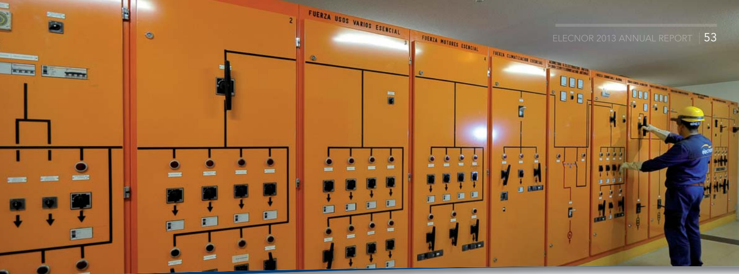
Maintenance of the Carmen y Severo Ochoa Hospital in Cangas del Narcea, Asturias
