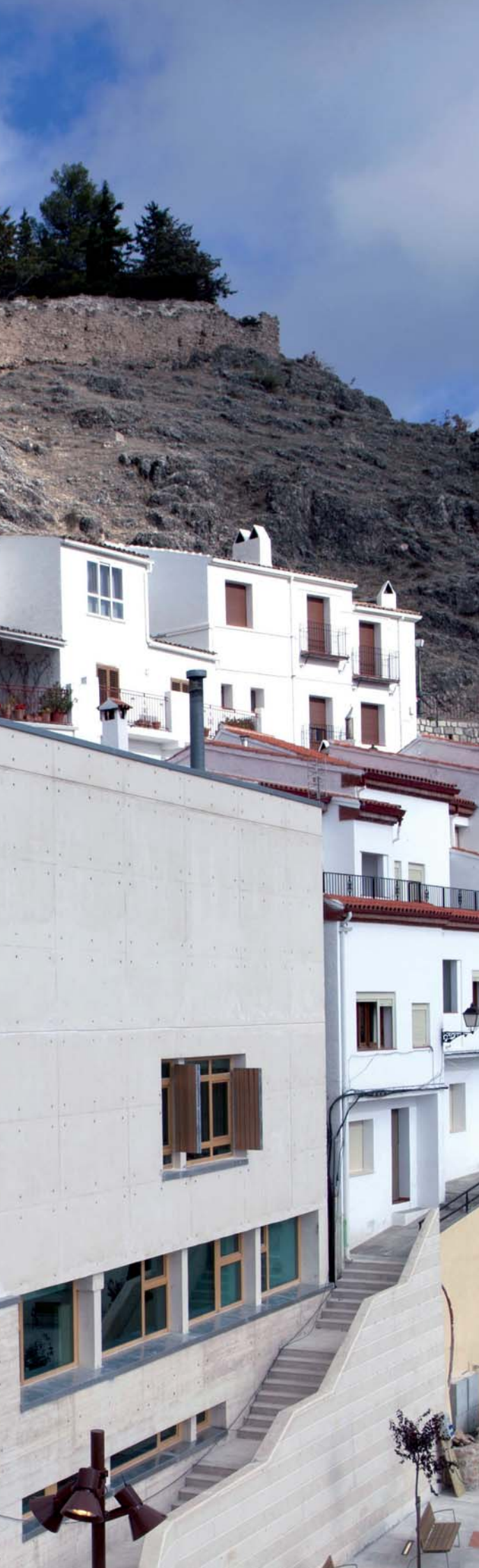
Refurbishment of the Segura de la Sierra council building in Jaen
