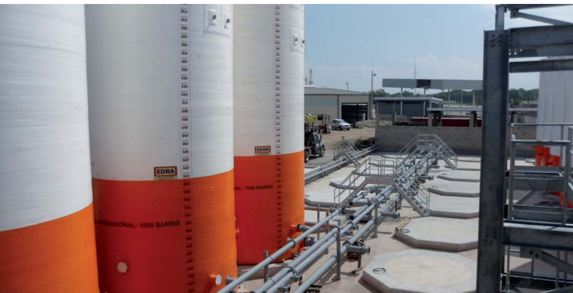
Construction of the Dos Bocas drilling fluids plant, Tabasco (Mexico)
