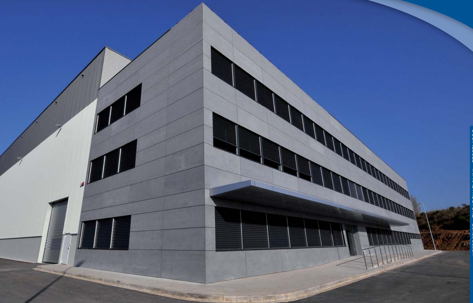
Construction of Audi Tooling facilities in Sant Esteve Sesroviros, Barcelona
