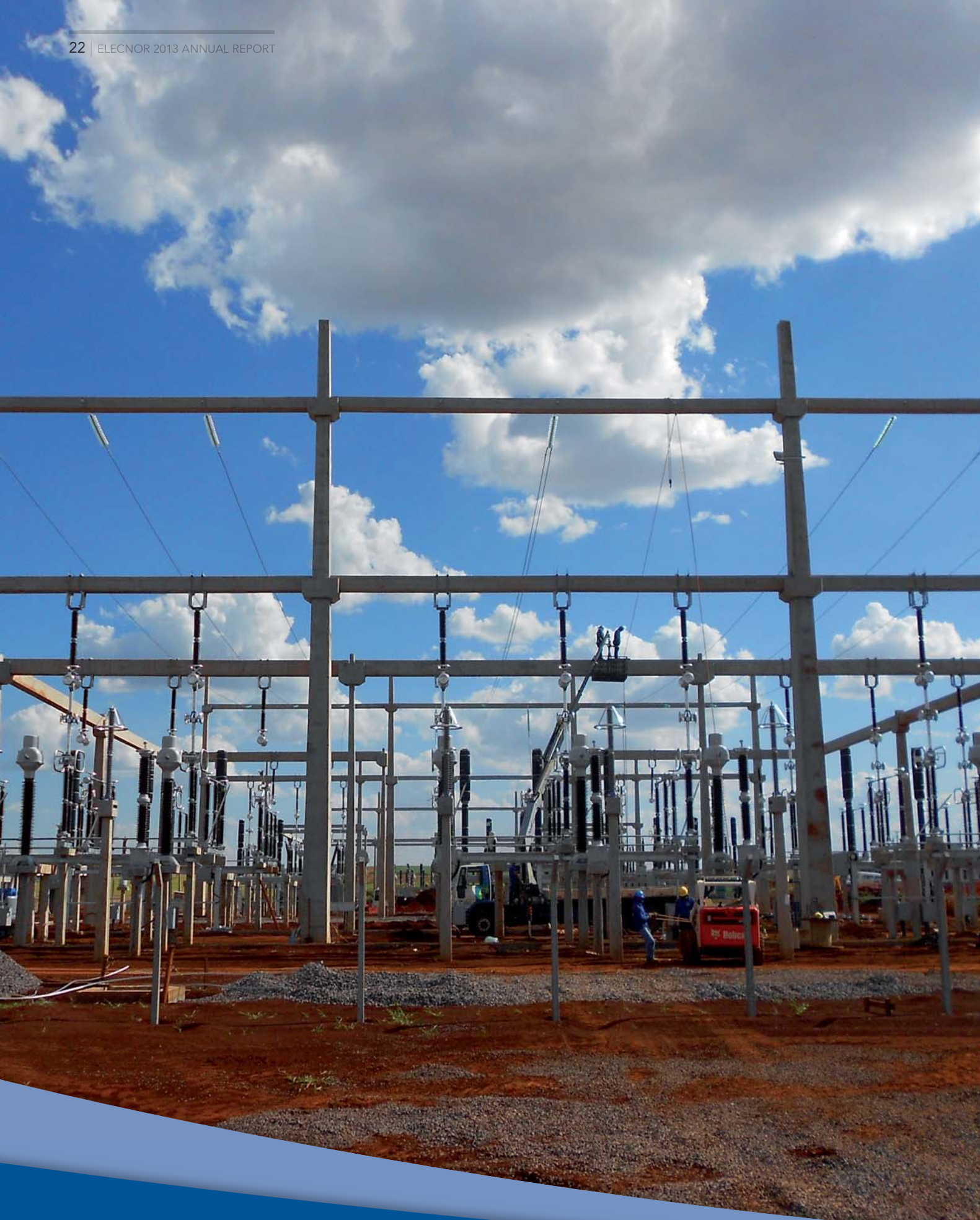
230 kV substation Cascavel Norte, Brazil
