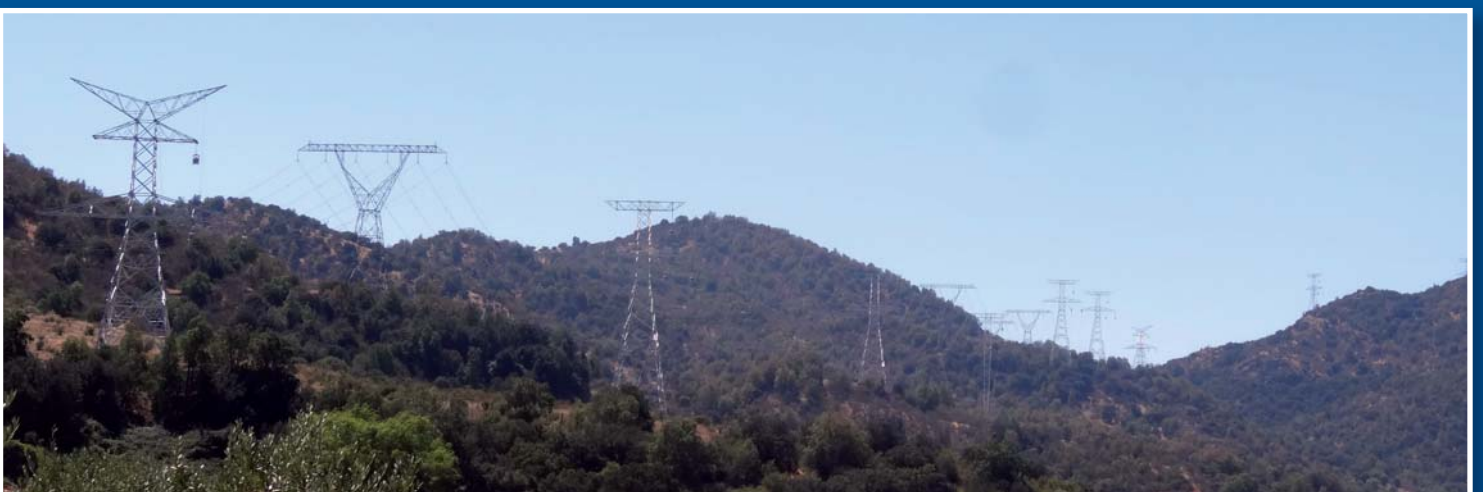
Ancoa-Alto Jahuel 2x500kV power line (Chile)
