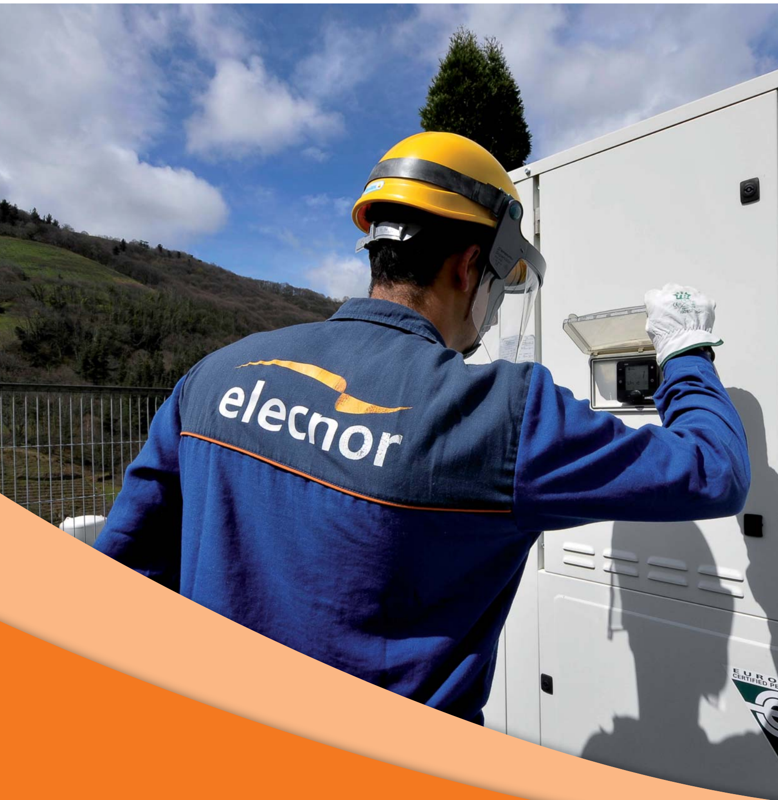
Maintenance of the Carmen y Severo Ochoa Hospital in Cangas del Narcea, Asturias
