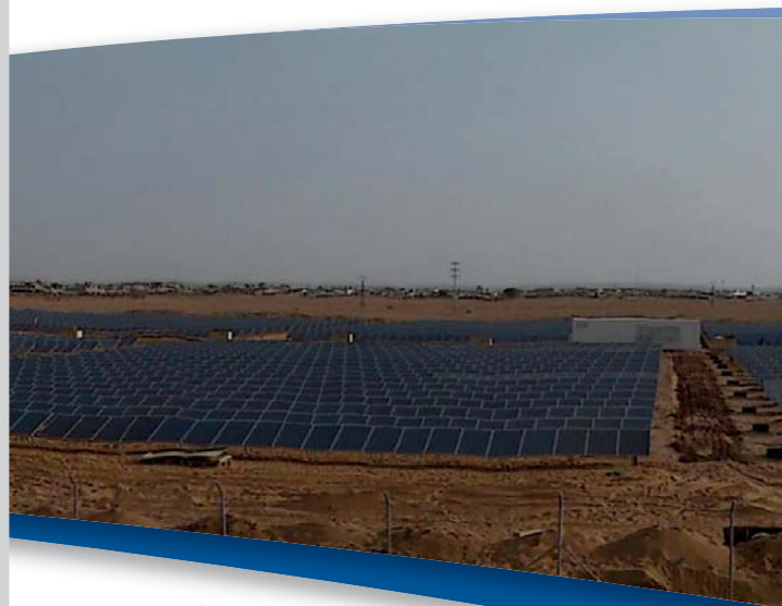
Zouerate solar PV plant (Mauritania)
