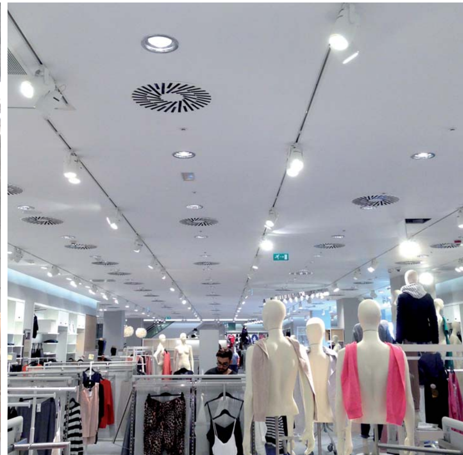
H&M installations at Nervión Plaza shopping centre (Seville)
