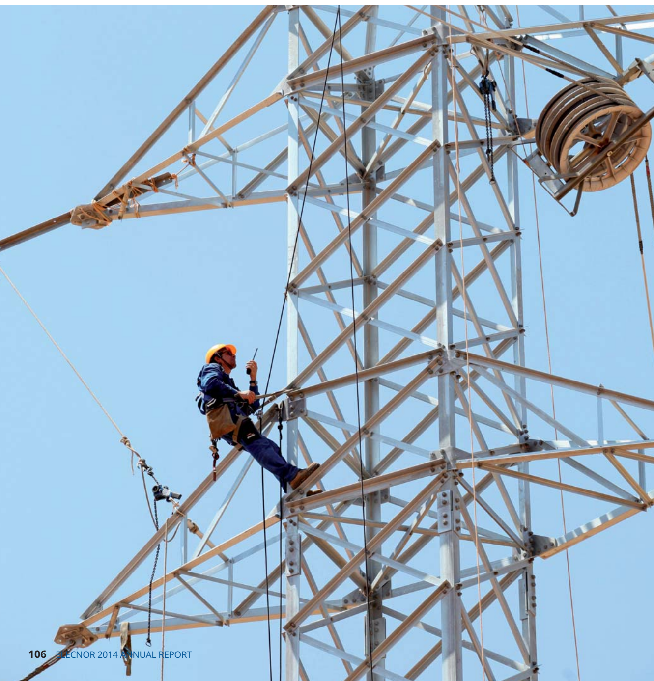
Alarcos-Piedrabuena 45 kV double-circuit, high-voltage aerial line (Madrid)
