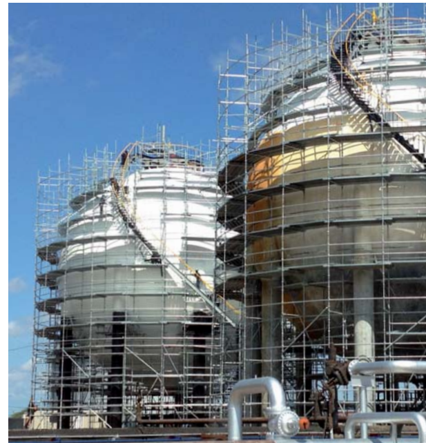
Anaco gas pipeline (Venezuela)
