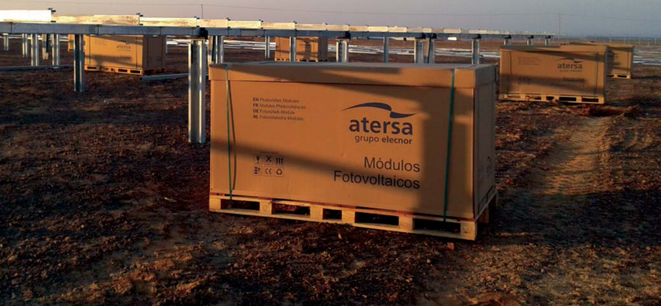
Azrak solar plant (Jordan)
