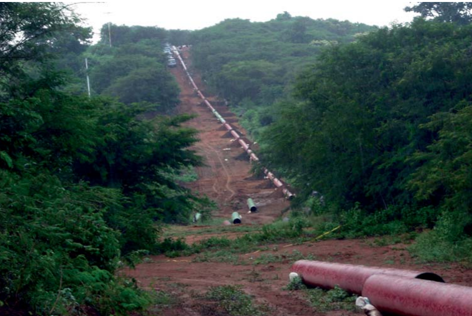
Anaco gas pipeline (Venezuela)
