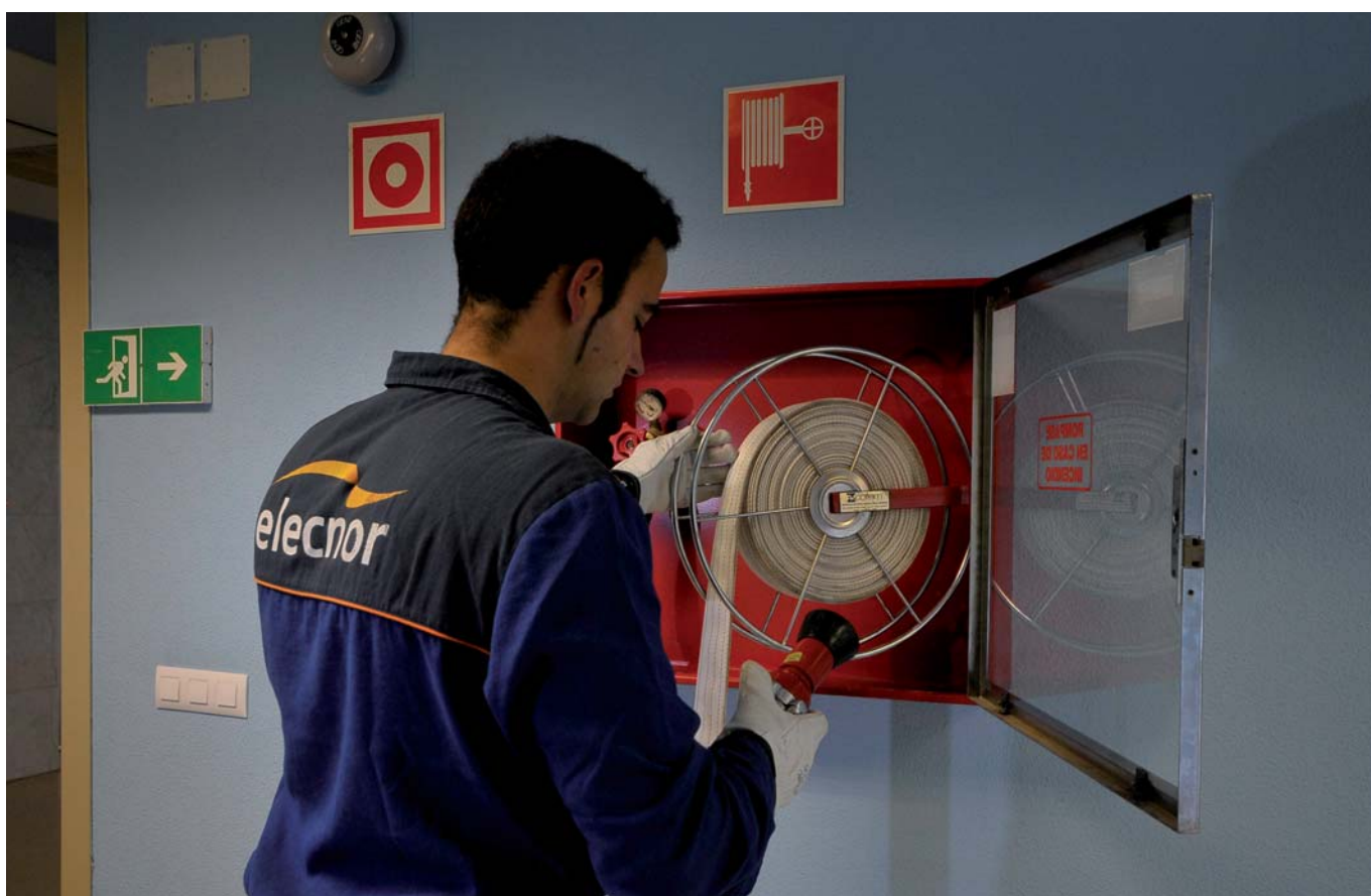
Maintenance of the Carmen y Severo Ochoa Hospital in Cangas del Narcea (Asturias)
