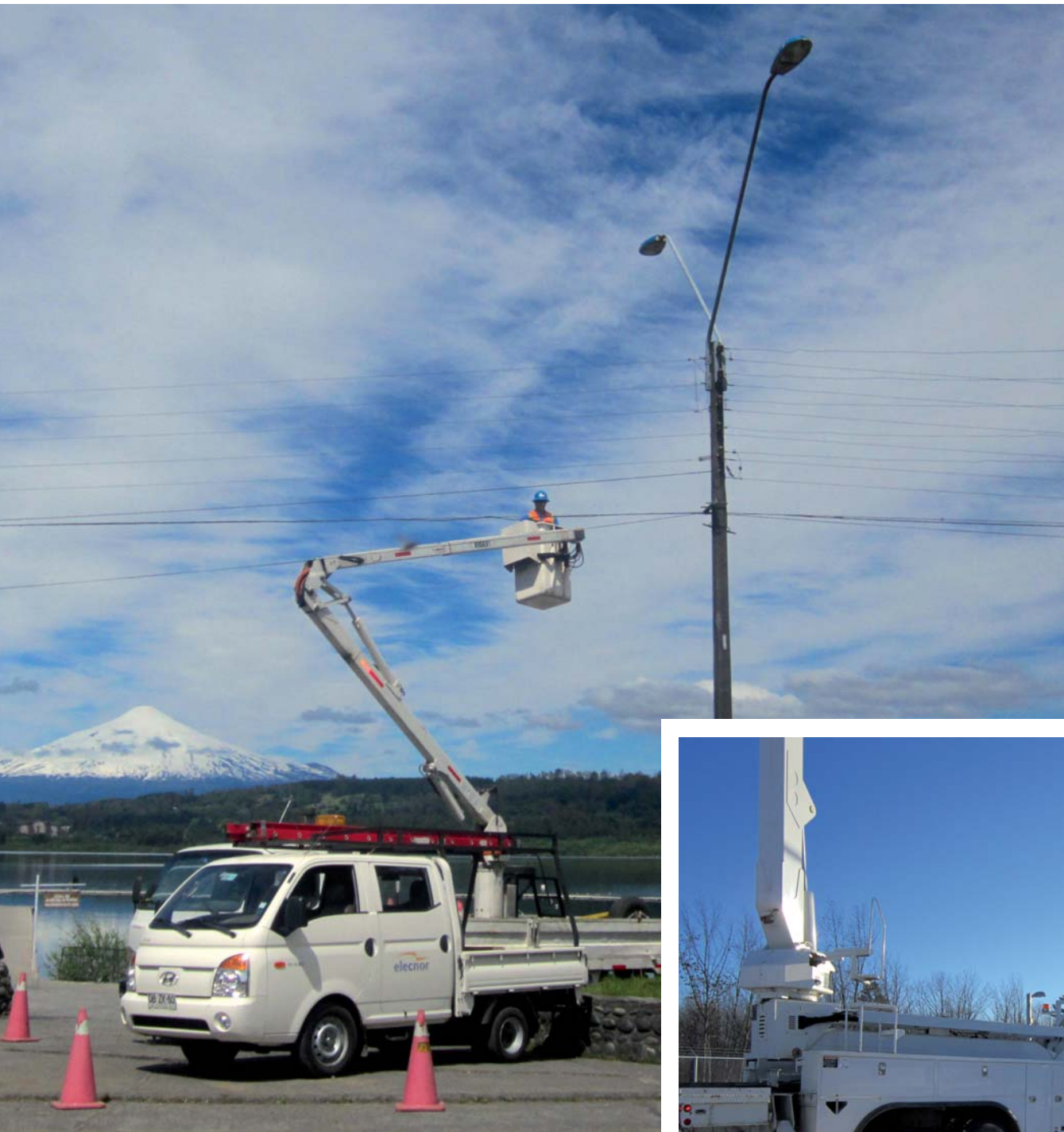
Public lighting in Villarrica (Chile)
