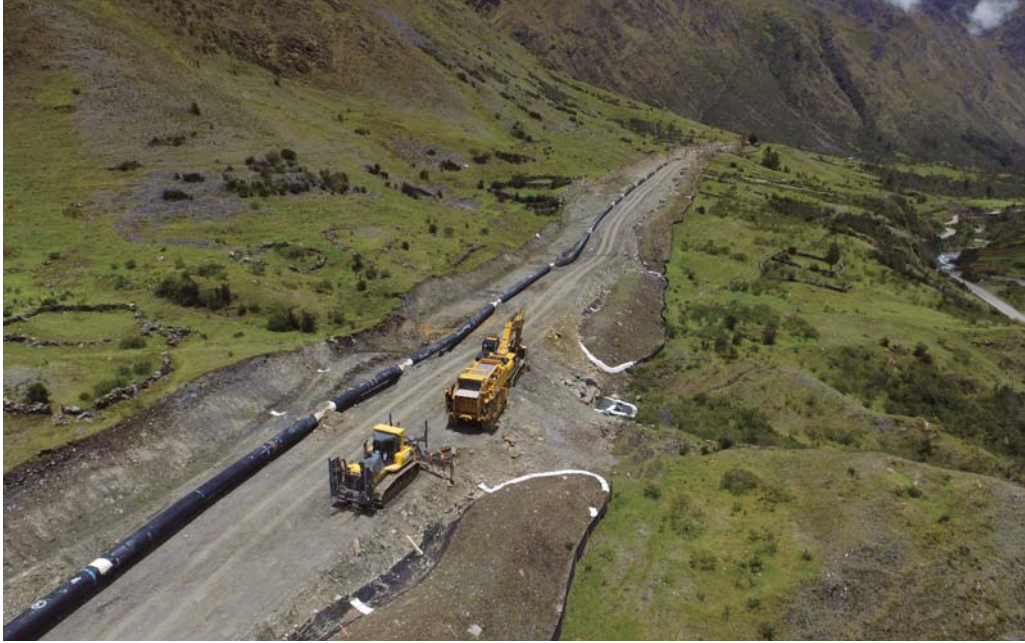
Southern Peruvian Gas Pipeline
