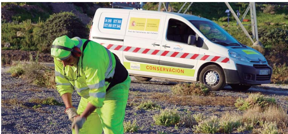
Environmental Services. Clearing vegetation by hand, Audeca
