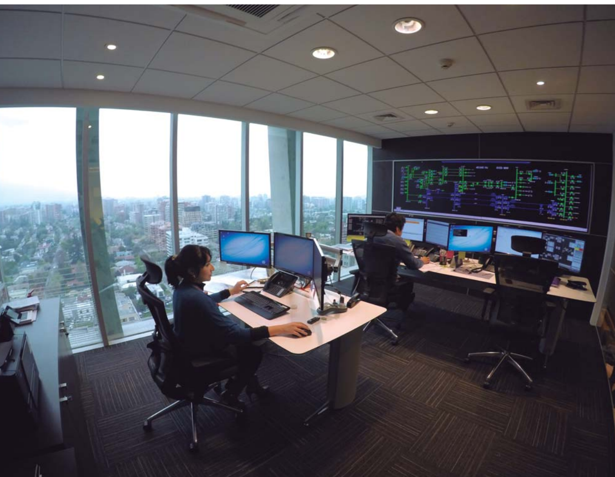
Control Centre in Santiago (Chile)
