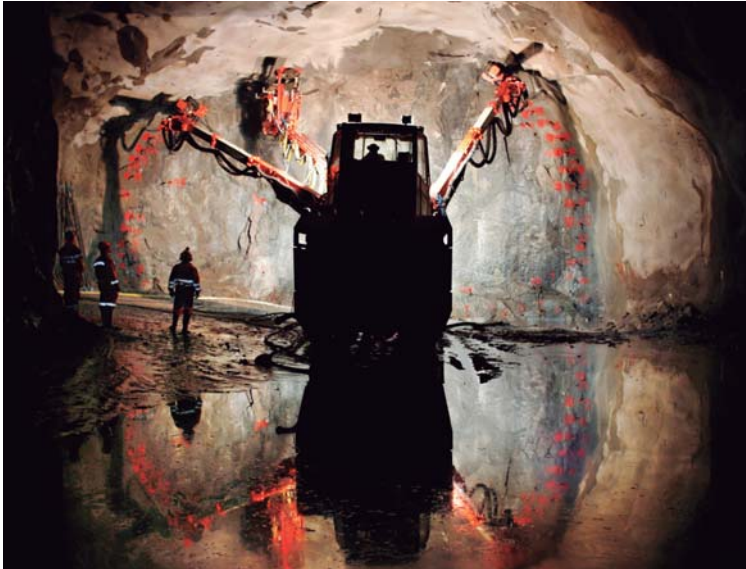
Follo Line railway tunnels (Norway)
