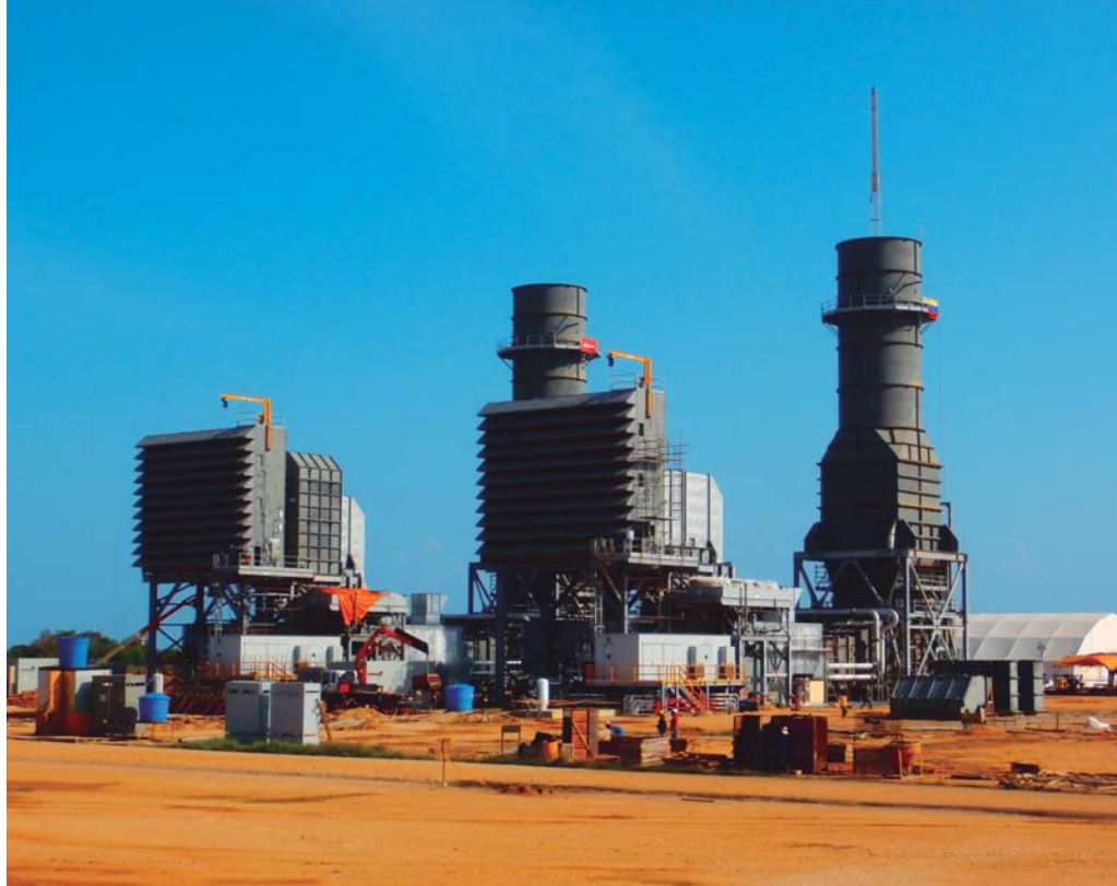
Water facilities at the Güiria Thermal Plant (Venezuela)
